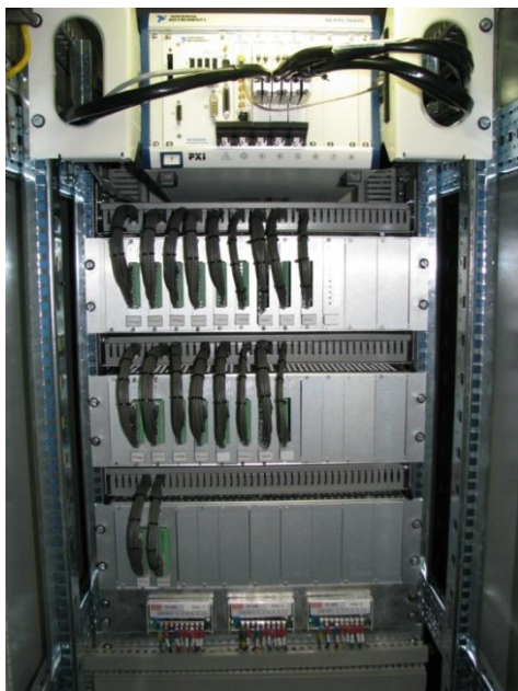
Figure 3: 11kV Substation PQ Monitoring Equipment
